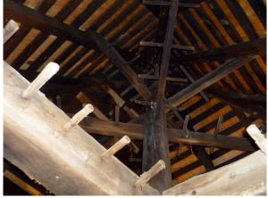
A typical farm smokehouse located in Middlesex County. Note the kingpost and beams studded with wooden pegs for hanging meat to smoke and age. Nails would rust in short order.
